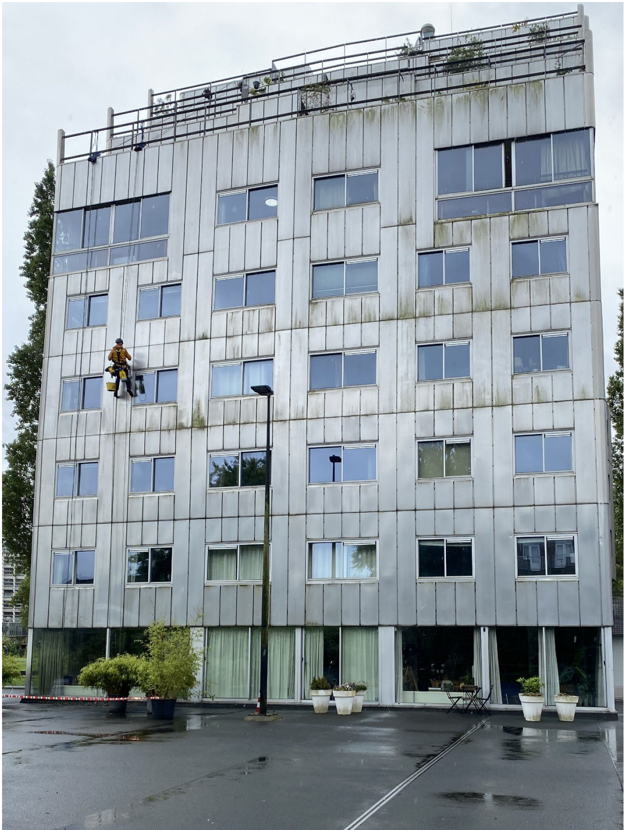
Cleaning the first lane of the north facade
