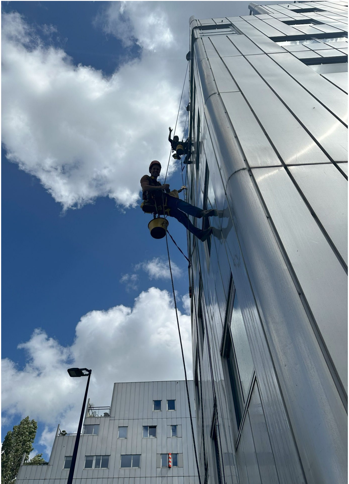
Building-Up in action cleaning the north facade
