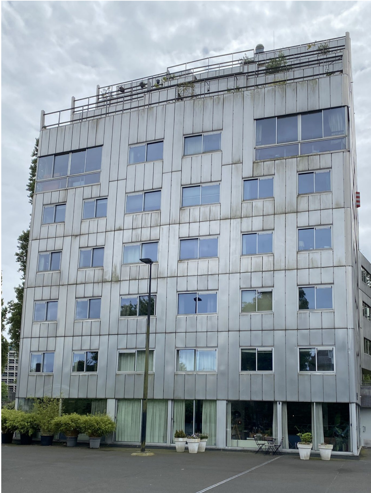
The north facade of Parktoren 2 in Amsterdam's Rietlandpark before cleaning
